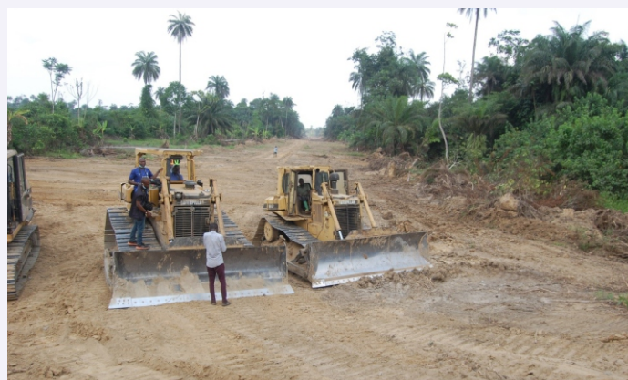
Construction Of Egbedi/ Amassoma Road
